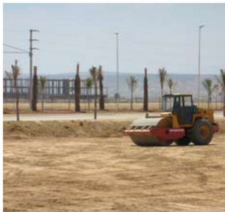
VVT-4: Groundworks underway (mid June 2008)
