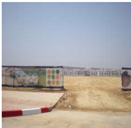
VT-5: Groundworks nearing completion
