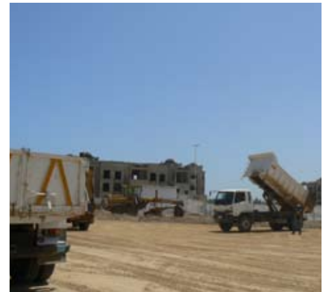
VVT-8: Groundwork completed and machinery arriving
