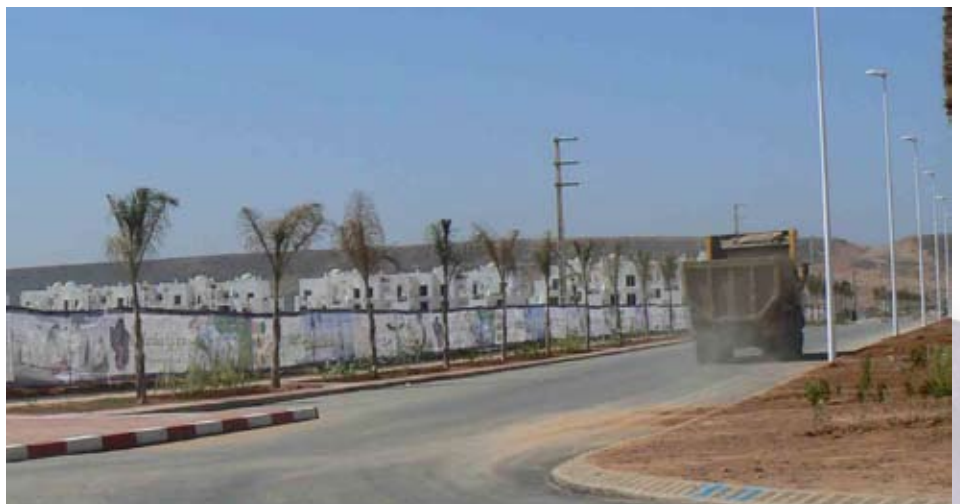
VVT-5 Site perimeter with mesh surrounds
